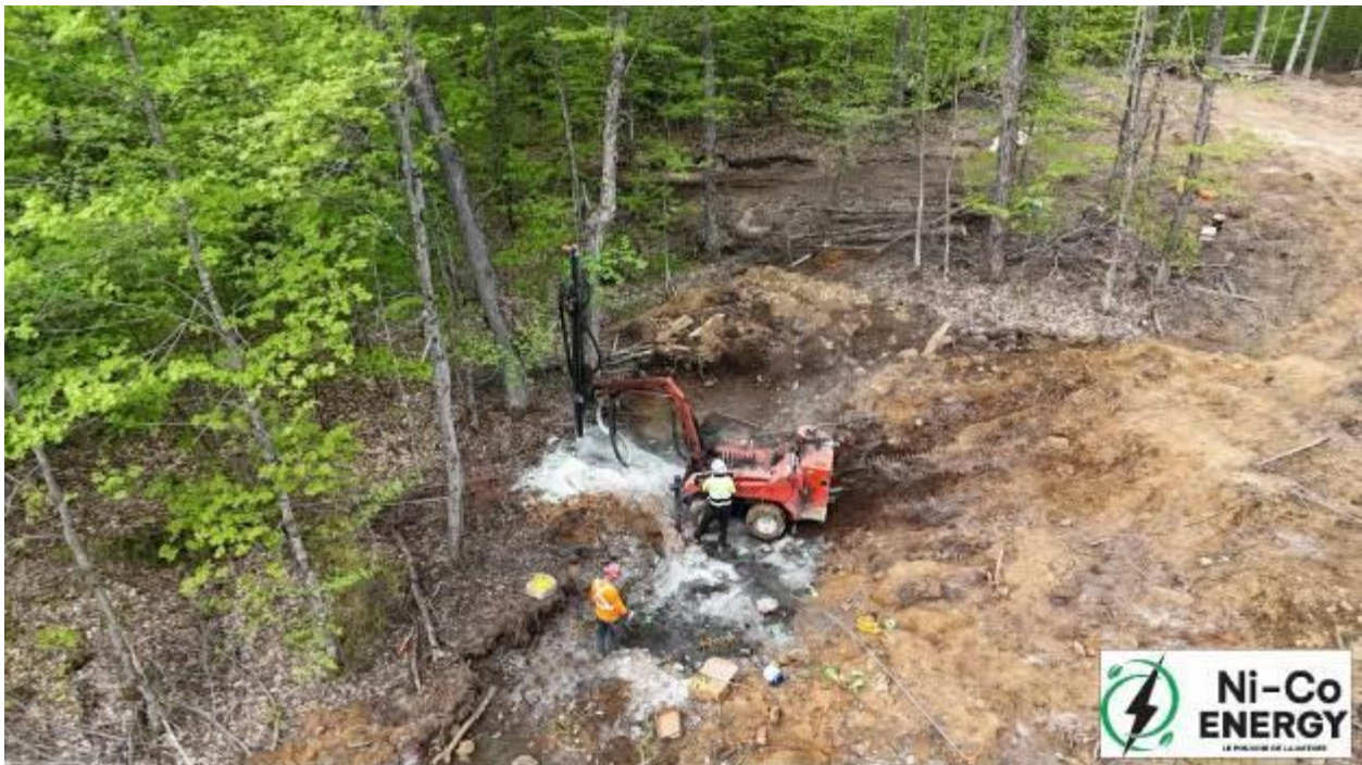
Stripping in progress
